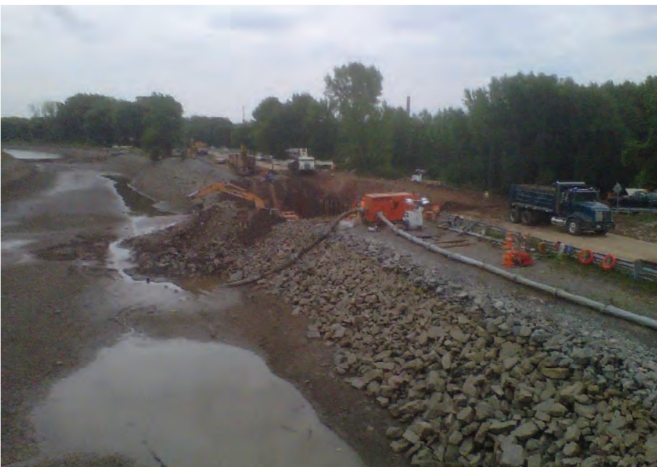
Figure T-20: Emergency repairs at the Erie Canal embankment in Albion, NY. (New York State Canal Corporation, 2012)
