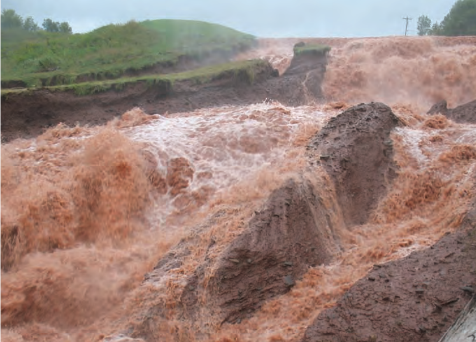
Figure L-25: Batavia Kill Dam No. 1 with flow through emergency spillway eroding downstream bank during Irene (NYSDEC, 2011)
