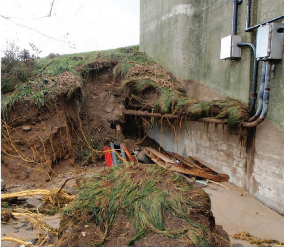
Figure T-17: Bridge scour at the south abutment of the Marine Parkway / Gil Hodges Memorial Bridge in the Rockaways. (MTA, Bridges and Tunnels, Adrian Moshe, 2012)
