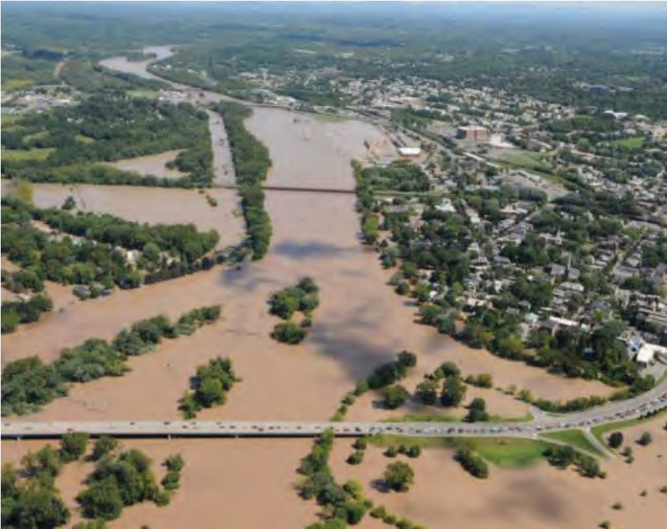
Figure T-19: The Hudson and Mohawk Rivers and other secondary waterways crested Monday, August 29, 2011. The storm impact in the Hudson Valley, Mohawk Valley, Catskills and Adirondacks was severe. (NYSDOT, 2011)
