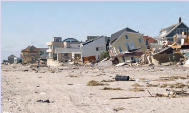
Figure L-03: Building damage in the Rockaways. (NYS DOS, 2012)
