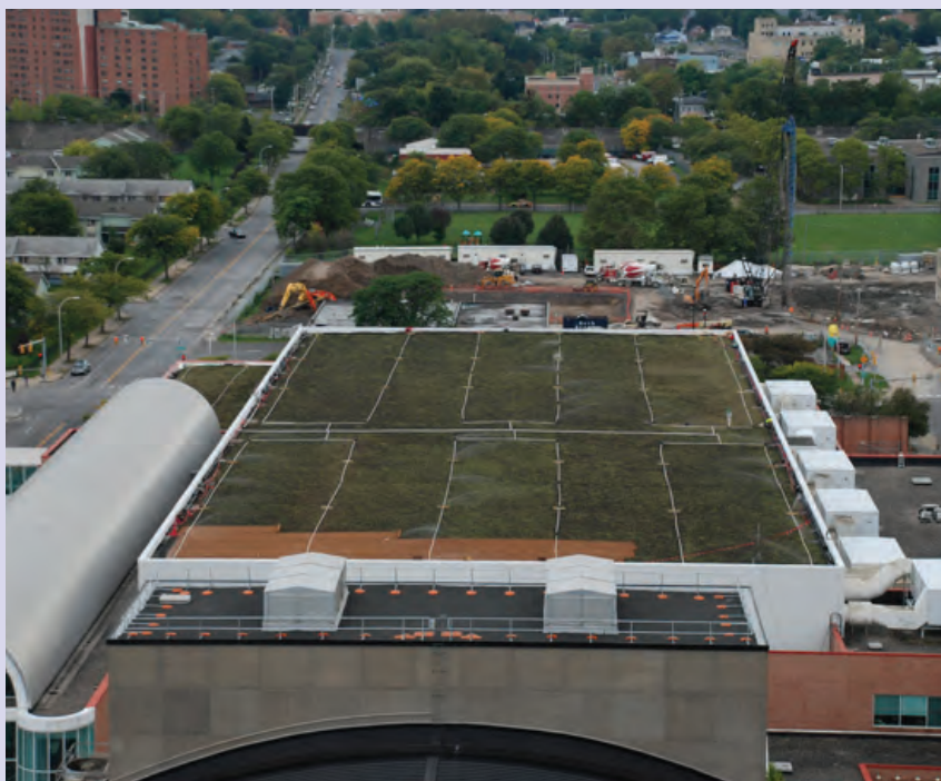
Figure L-24: Large green roof installed at “OnCenter” in Syracuse is a major project of the “Save the Rain” Program (Onondaga County, 2012)
