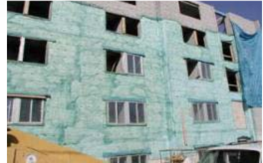
FLUID-APPLIED SPRAY FOAM
