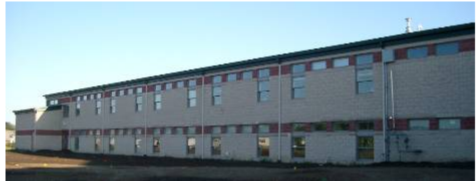
North side of classroom wing
