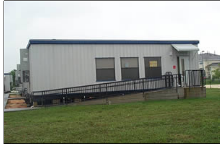
FL Control Unit
