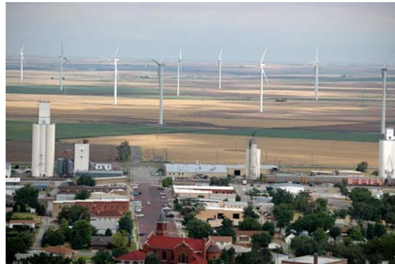
Kansas' newest commercial wind farm is the Spearville Wind Energy facility – a 100.5 MW wind farm that went online in September 2006. Photo courtesy of Phil Duncan, KCP&L
