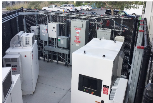
EVgo 30 kW / 50 kWh 2 nd life batteries for DC-fast charging application
