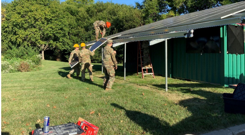
Camp Dodge soldiers packing up crate: removing PV panels
