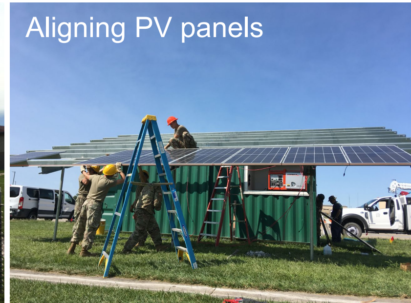
reassembly at Camp Dodge, note 48" anchors
