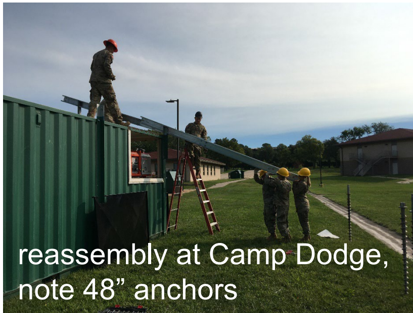
Aligning PV panels
