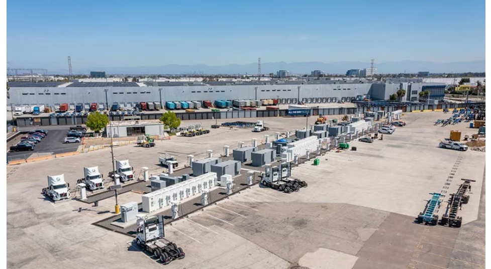
A 9 MW microgrid charging solution near the Port of Los Angeles. Capable of charging 96 EV trucks simultaneously. Owned by Prologis to serve Maersk's drayage truck fleet.
