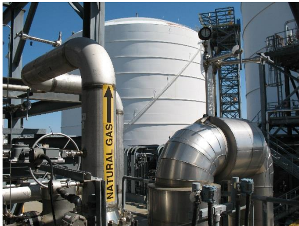
Distrigas facility, part of GDF SUEZ NA
