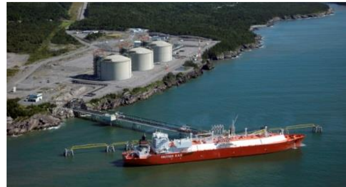
Canaport LNG. Photo courtesy of Repsol
