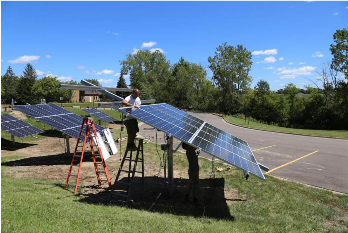
The Michigan Agency for Energy and the Michigan Public Service Commission were the first state agencies in the country to make energy improvements to their properties using PACE. This project, which was privately financed, included the installation of a small solar array, LED lighting, and variable speed pumps for heating and cooling. Photo courtesy of Lean and Green Michigan.
