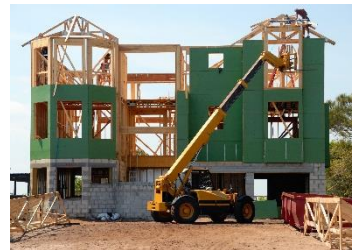
New construction and existing building retrofits
